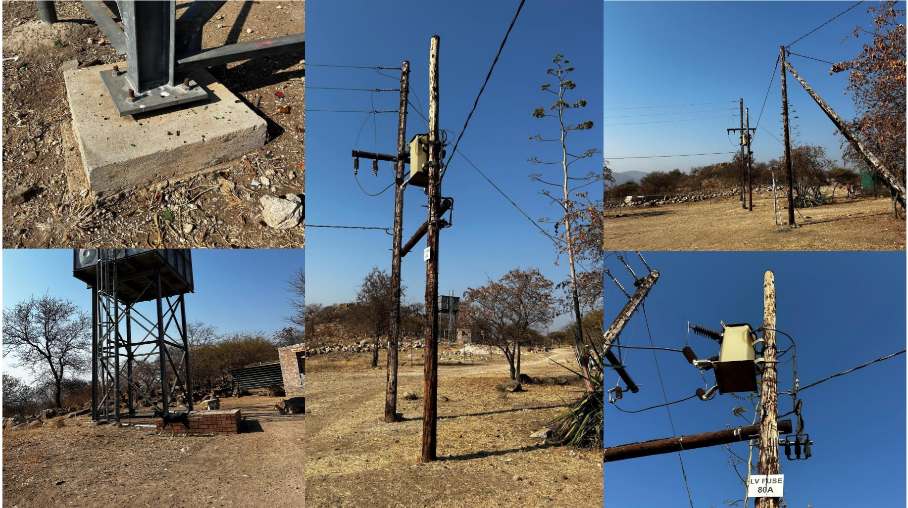
Photos 1: Infrastructures, Powerlines and water tank stand (about 595,1m East of the South Shell Pit)
